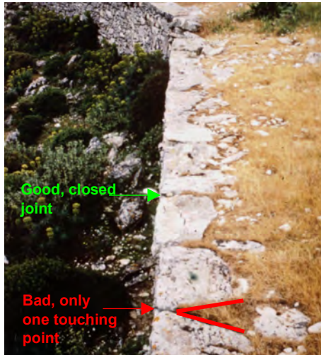
figure 23: joints between topstones
