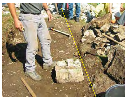
figure 7: laying the foundation
