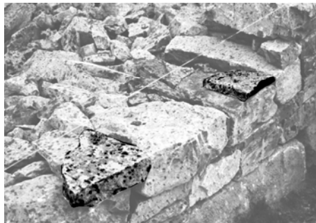
figure 13: stones used to equalize the height adjacent stones
