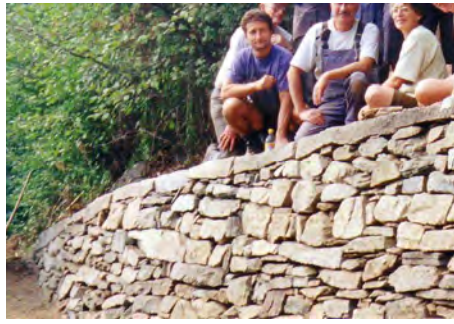
figure 18: topstones placed horizontal
